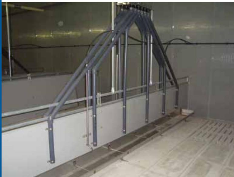
The charging of the hoppers through automatically controlled valves. When all Feed Distribution Units are filled the central pneumatically controlled opening mechanism opens all units for simultaneously feeding in all sections.
